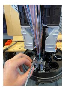
• Place the screws into the metal plate then wrap the binding strings around the screw to ensure the ribbon cable into position.
