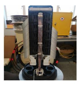
• Rotate the loop manager back into the closure. Being careful not to strain the elements.
