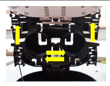
• Cross the fibres at the bottom and route the fibre up to the tray which is to require the splitter.
