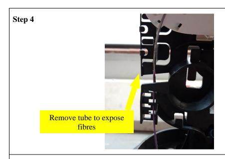
• Remove the tube to expose the fibres at previously marked point using approved practices.
