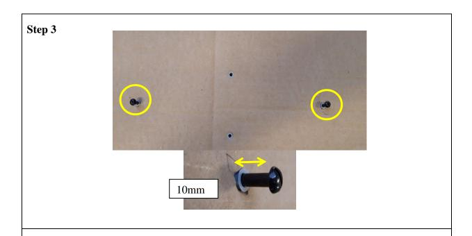
• Screw the 2 screws as shown into the wall plugs and leave the screw head approx. 10mm from the wall face.
