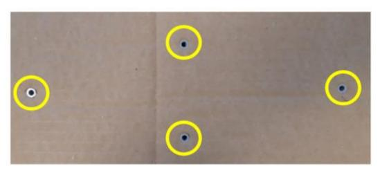
• Drill 4 holes as marked using the 5mm drill bit and fit wall plugs into the holes.
