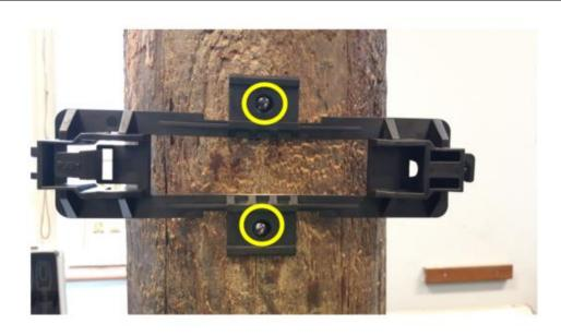
• Screw bracket to pole using screws provided.
