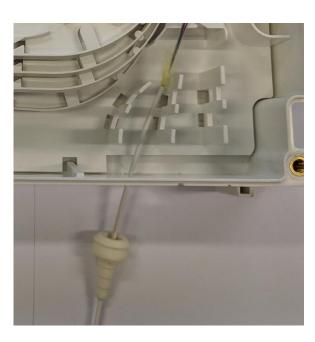
• Remove cable outer sheath to expose approximately 1.5m of fibre. Insert the cable through the Cable Grommet and into box.
