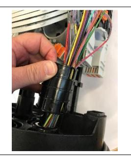
• Slide the tool over the gland and push into the base. When clips disengage remove gland from base and carefully pull out all tubes and fibres.
