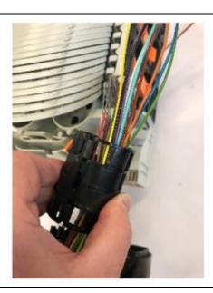
• Snap the 2 halves of the gland removal tool around the tubes.
