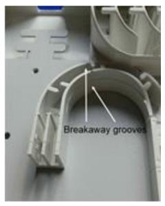
• The fibre guide supplied with the MDU internal splitter node incorporates breakaway grooves. This enables the left-hand side of the guide to be snapped off enabling installation of loop kit.
