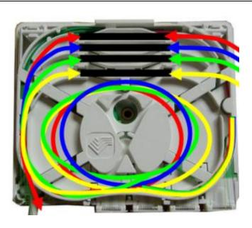
• Simultaneously coil the all the excess fibers lengths from one side of the splice protector in the central area of the tray.
