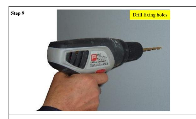
• Drill the holes using a drill and a 6mm drill bit.
