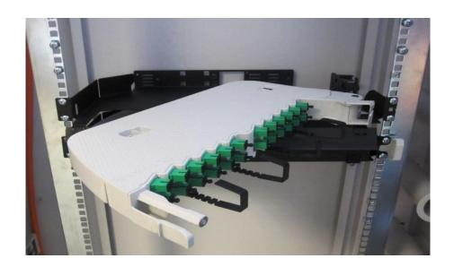
• Replace the protective cover over the splicing area by sliding the right-hand clip into position and then pushing firmly down until the left-hand clip is secure.
